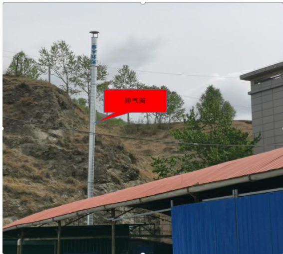
喷漆房排气筒
